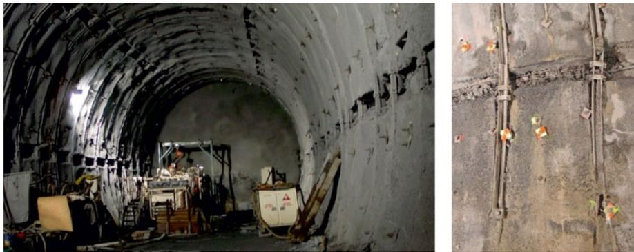
**Figure 2.32.** Left: Support class ES6A of the Lötschberg Base Tunnel (eastern tube at km 28'759; [36]); right: buckled steel ribs (eastern tube at km 30'421; [37]).
