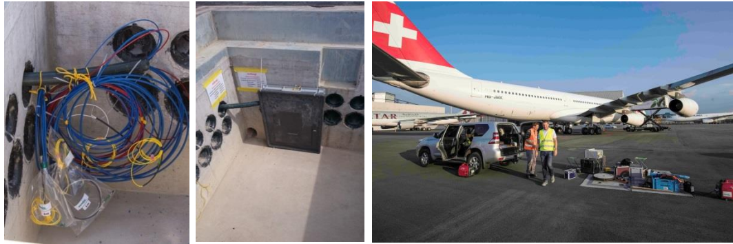
Fig. 124 Cable ends in the electro shaft directly after installation (left) and stored in access box (right) after packaging
