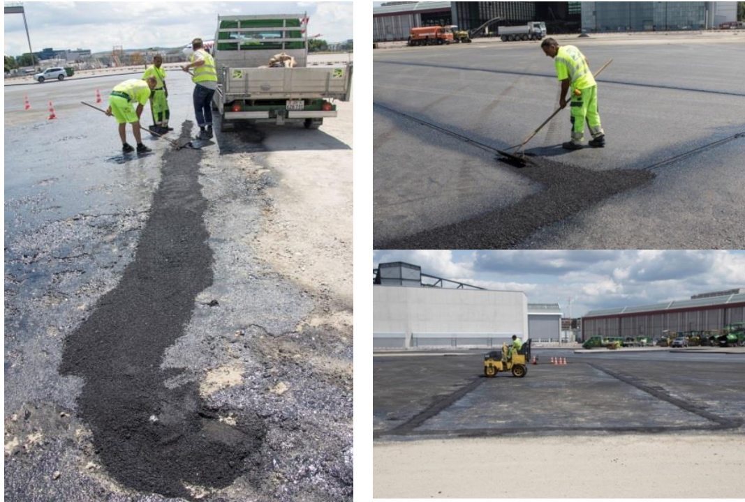
Fig. 45 Covering of the sensors with fine asphalt (left and top right); small compactor passing over the covered sensing cables (right) at Zurich Airport test site
