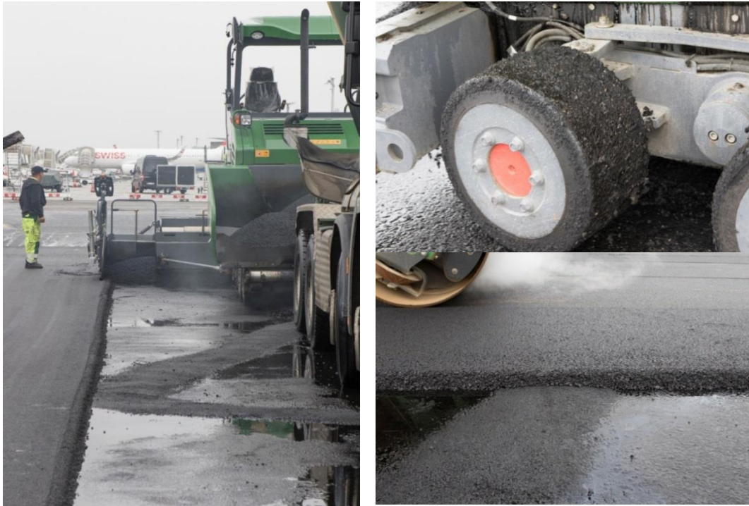
Fig. 46 Paver passing over the sensor (left); wheel of a paver with gravel sticking on it (top right) and passing of a heavy compactor over the asphalt layer and the sensors (bottom right) at Zurich Airport test site
