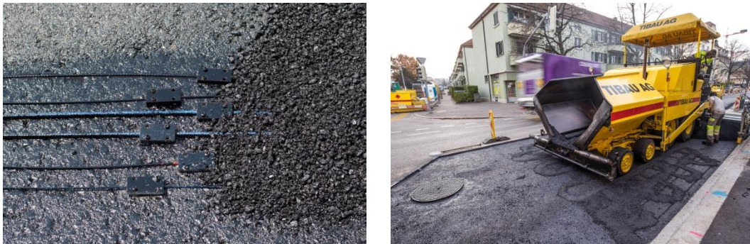
Fig. 43 Covering of the sensors with fine asphalt at Zurich Airport (left); asphalt paver passing over the covered sensing cables (right) at Hohlstrasse test site
