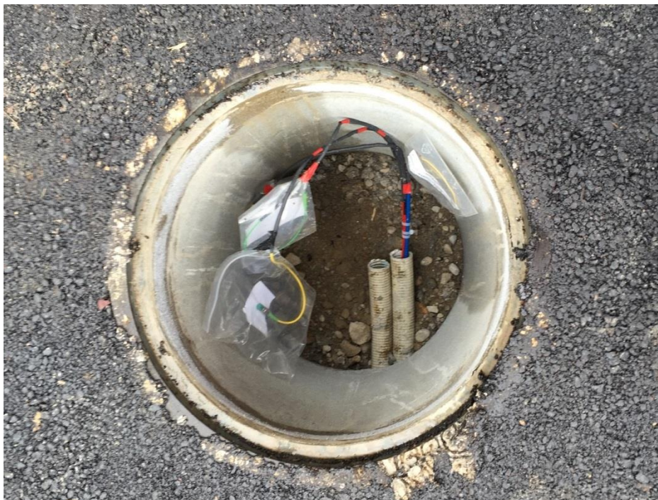
Fig. 51: Cable shaft at Hohlstrasse test site with short cable ends
