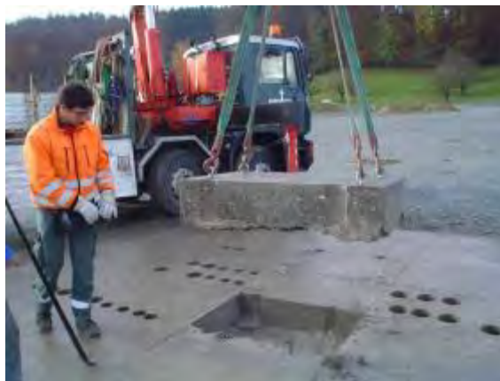
Fig. 5.70 Pulling out of one of the pavement blocks
