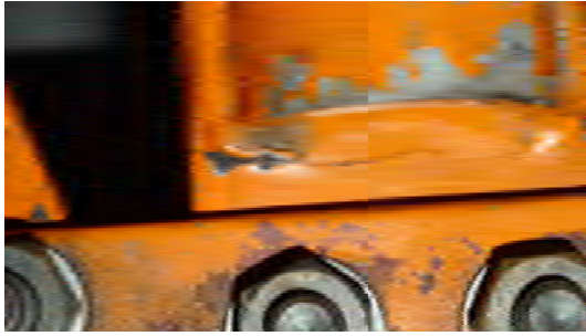
Fig. 6.6 Crack in a strut connection
