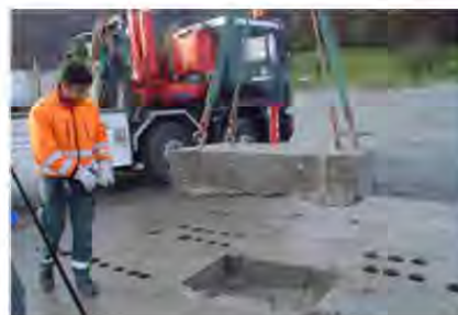
Figure 8. Extraction of asphalt slab from test pavement.
