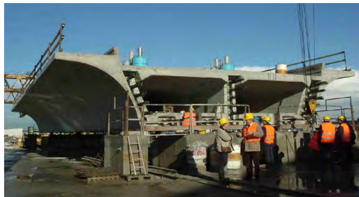
Figure 16: Piacenza viaduct anchorage and transparent stocking area [23] Figure 17: Piacenza viaduct full span precast deck in anchorage and transparent stocking area [23] cap [18].
