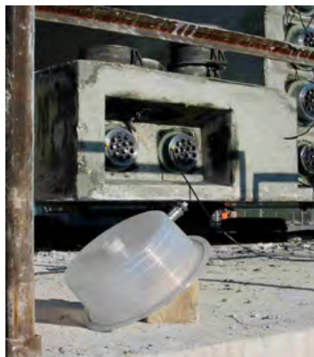
Figure 16: Piacenza viaduct anchorage and transparent stocking area [23] Figure 17: Piacenza viaduct full span precast deck in anchorage and transparent stocking area [23] cap [18].
