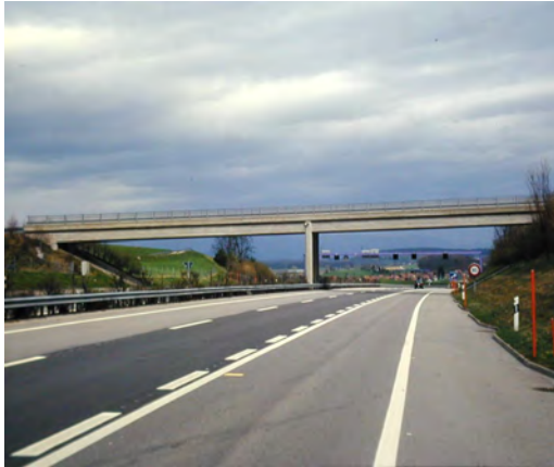
Figure 25: Flyover “Pré du Mariage” near Avenches (highway A2 Switzerland)
